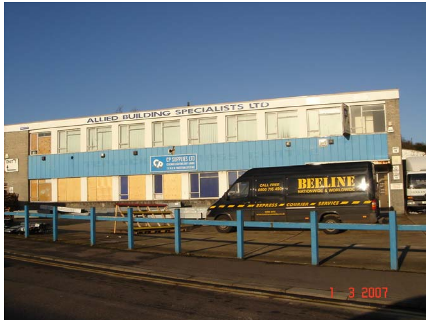
Previous building on site
